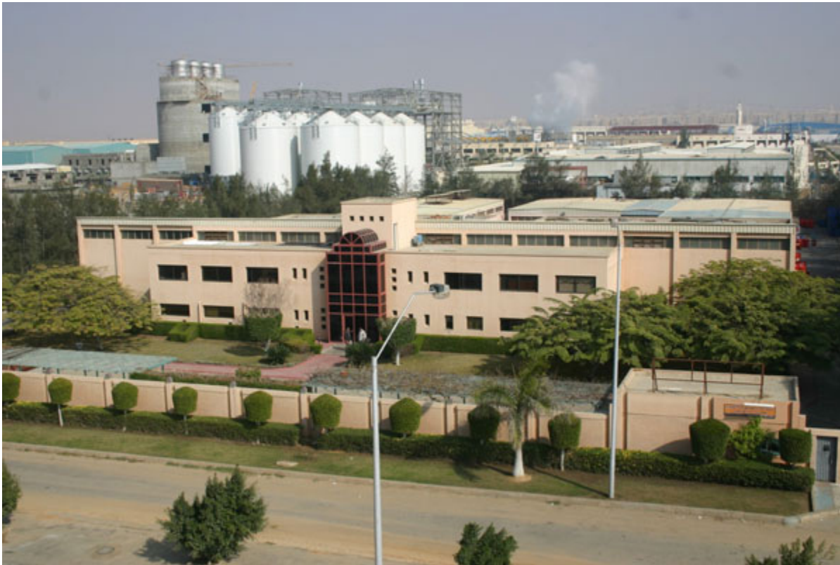
Figure 1. SwissChem Factory in 6th of October City, Western Cairo, Egypt
