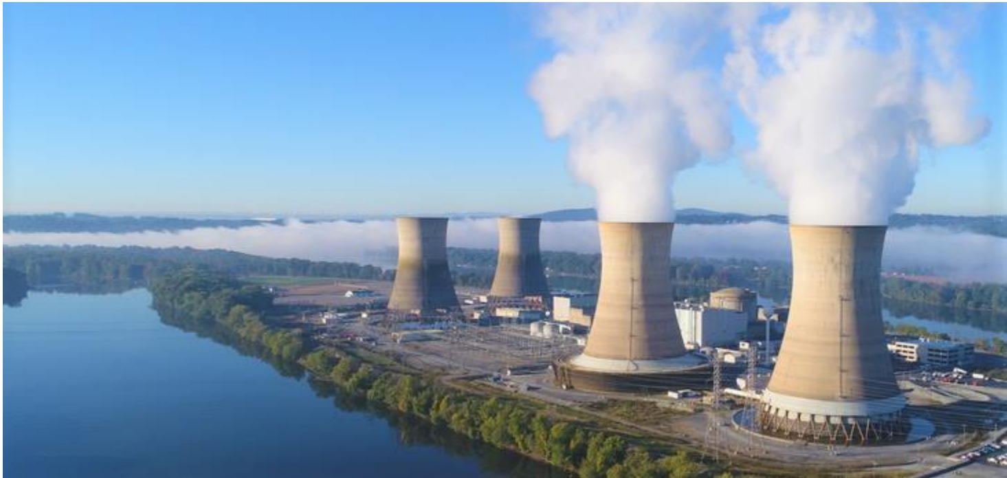
Dresden generating station in Morris, Illinois
