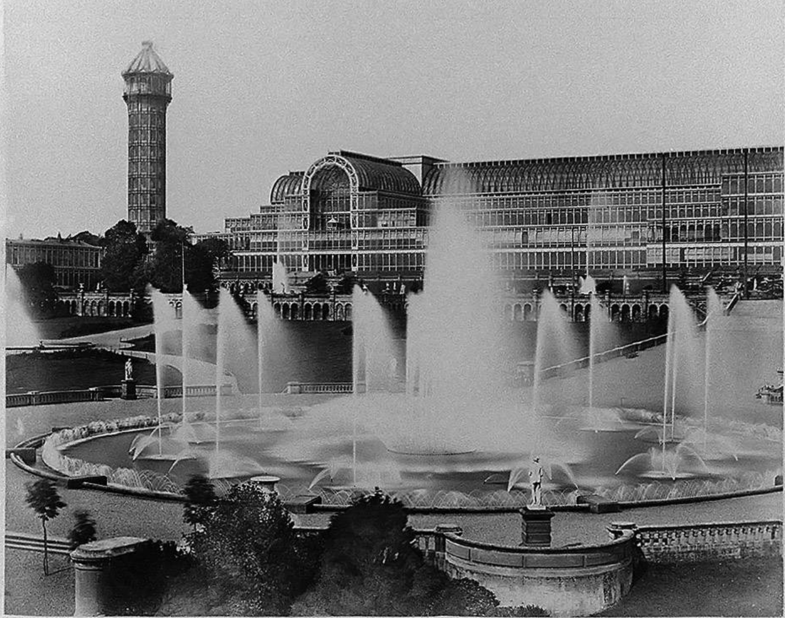
South Transept & South Tower
